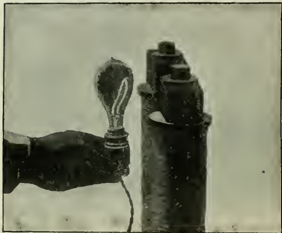
FIG. 5.—TRANSMISSION OF MAGNETIC FORCE ACROSS A VACUUM.
